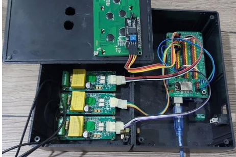
GAMBAR 2. PENKABELAN INSTALASI SENSOR PZEM-004T
